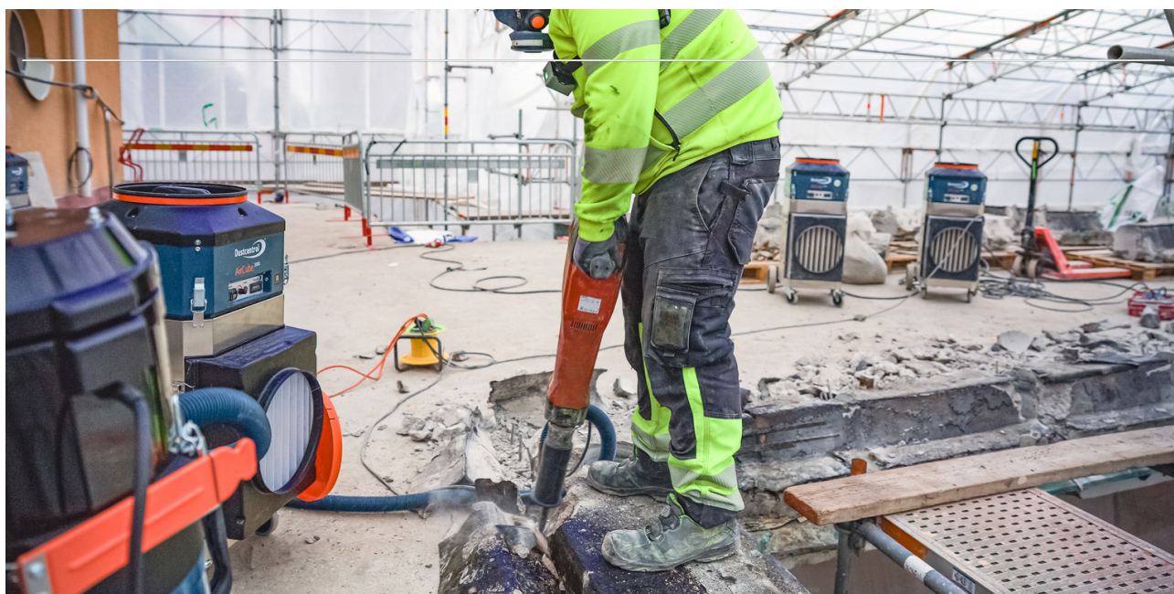
Demolition and renovation – where the dust is worst and the filter works hardest.
